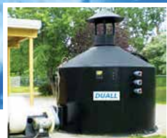
Carbon Canister with Integral Fan
