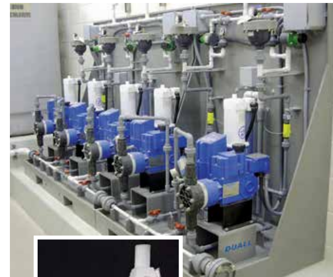
Self-Contained Chemical Feed Skids
