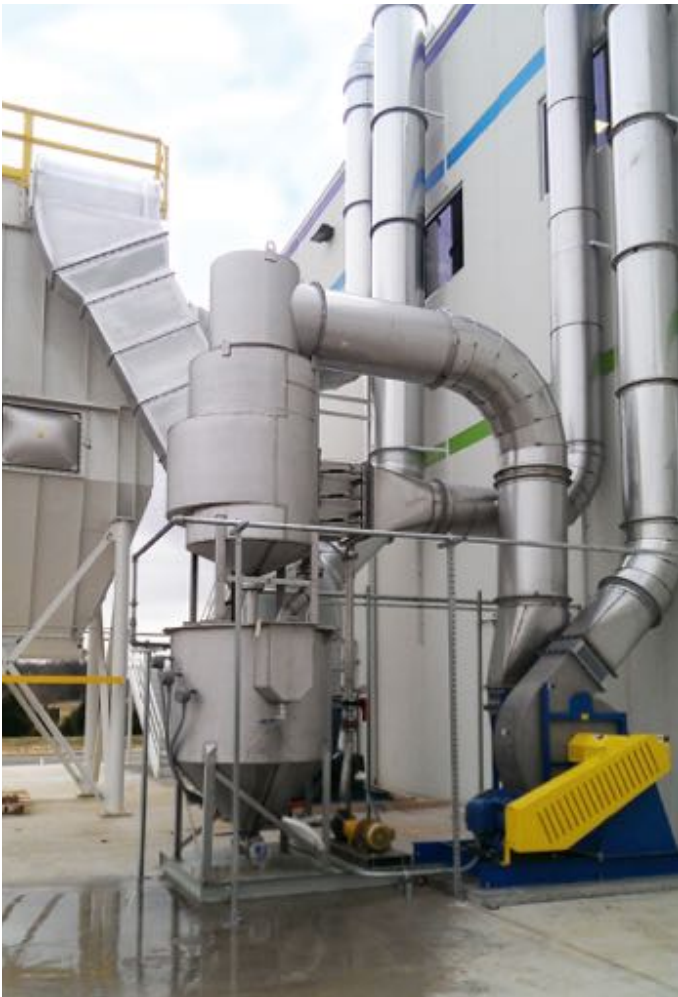
Figure 2. Scrubbers are pollution control devices that use liquid to wash unwanted pollutants from a gas stream, or that inject a dry reagent or slurry into a dirty exhaust stream to ‘wash out’ acid gases. Scrubbers are one of the primary devices that control gaseous emissions, especially acid gases.
